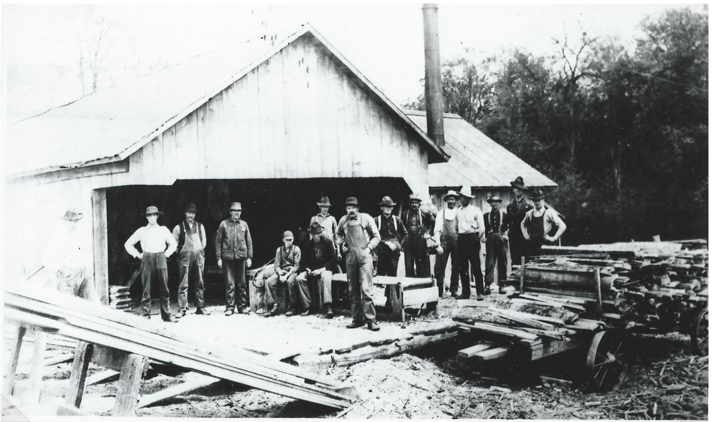
Peter Johnson's saw mill crew.
