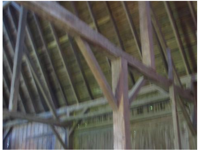
Traditional Post and Beam Construction in the Barn Next Door You can see the axe marks on the hewed beams.
