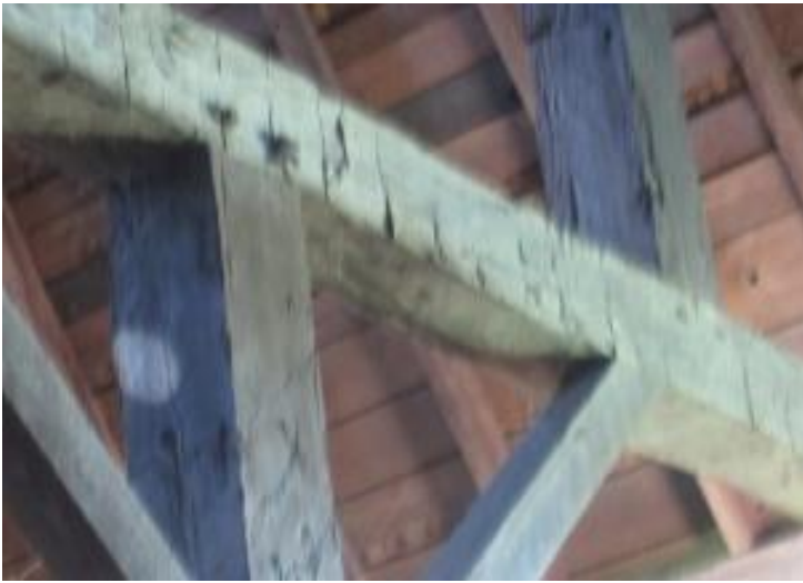
Traditional Post and Beam Construction in the Barn Next Door You can see the axe marks on the hewed beams.
