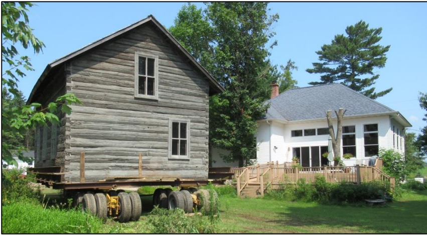
Meanwhile back at Liberty School the process began to get the log building ready to move out. Our Yesterday House was jacked up and sets of wheels were put underneath the building. Long iron beams were in place in both directions to keep the building level as it was jacked up.
