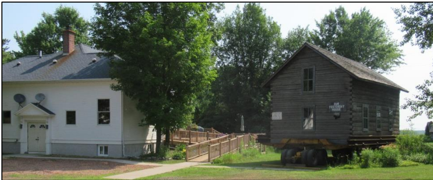
Meanwhile back at Liberty School the process began to get the log building ready to move out. Our Yesterday House was jacked up and sets of wheels were put underneath the building. Long iron beams were in place in both directions to keep the building level as it was jacked up.
