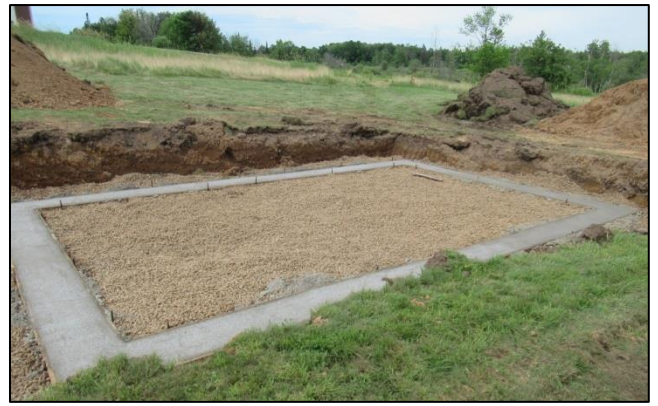
A cement footing was poured and loads of rock were brought in to fill inside and out.
