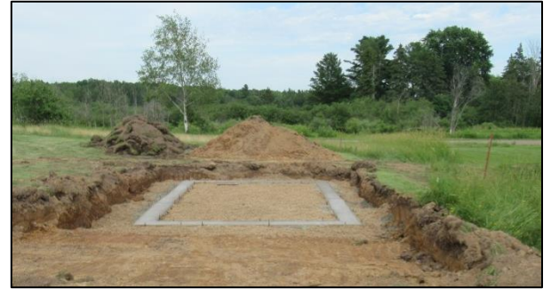
A cement footing was poured and loads of rock were brought in to fill inside and out.
