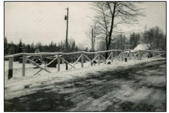
Jacob built this beautiful birch fence on the south side of the Hwy. 102 curve coming down to the lake.
