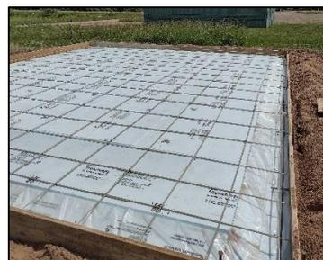
Reinforcement bars were placed above the Styrofoam in a grid pattern --- and the site was ready for concrete.
