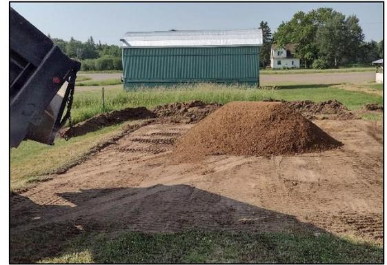
After the top soil was removed four loads of sand were brought in to make a level base for the concrete slab.
