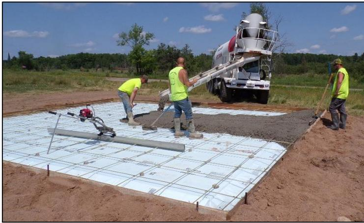
The pouring of concrete was delayed because of hot weather. Two loads of concrete were delivered and poured over the Styrofoam to make a great new floor for our Machine Shed.
